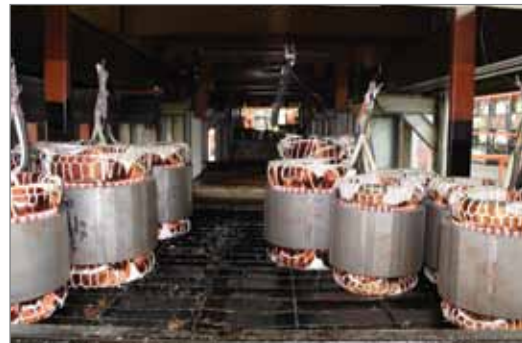
Automatic Impregnation Plant
